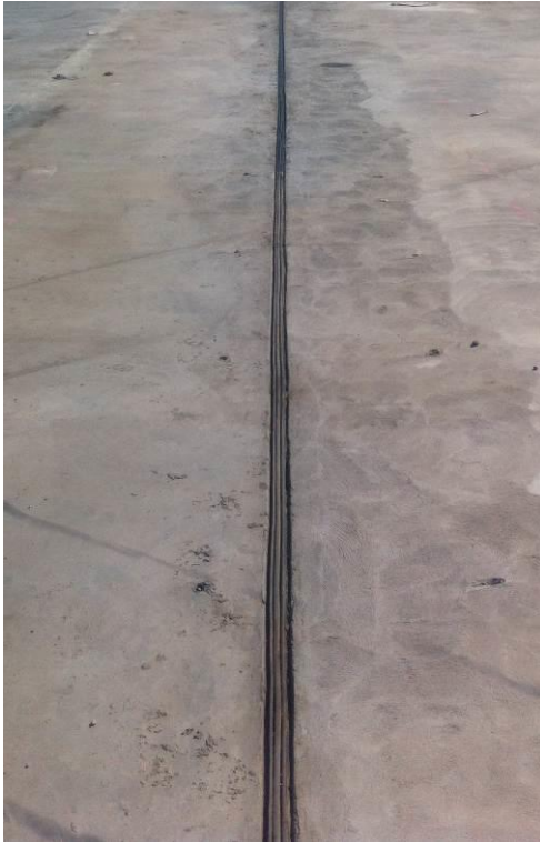
Wizflex between concrete deck
