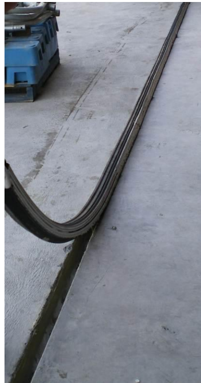
Wizflex into warehouse slab
