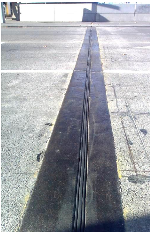
Wizflex between Silspec 900 PNS
