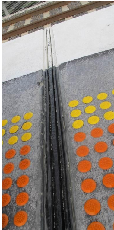
Wizflex on Railway Station Platform
