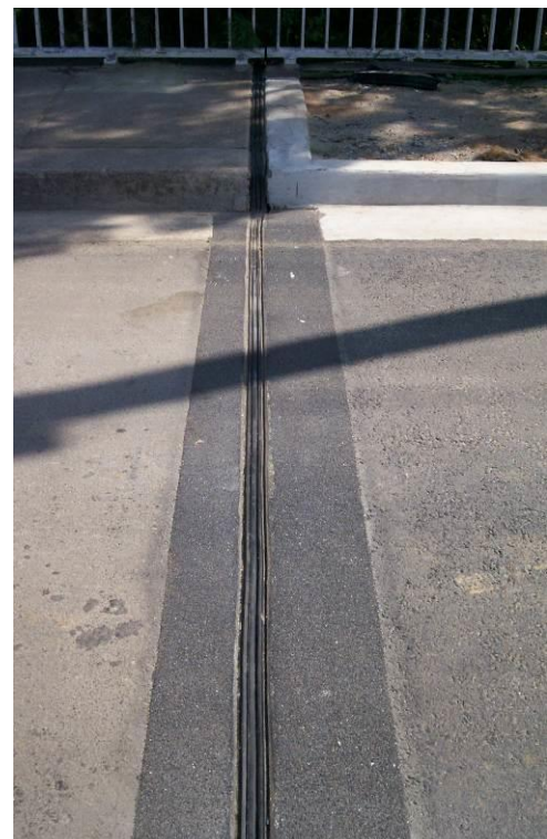
Wizflex between Silspec 900 PNS
