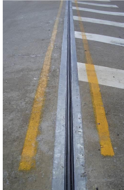
Wizflex between steel angles
